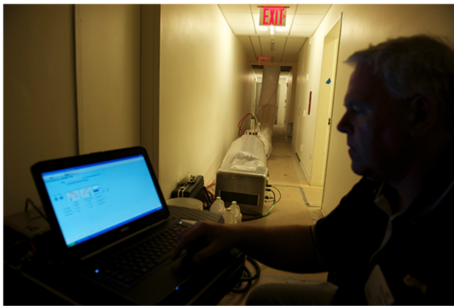
A technician monitors the computerized duct-sealing process.
